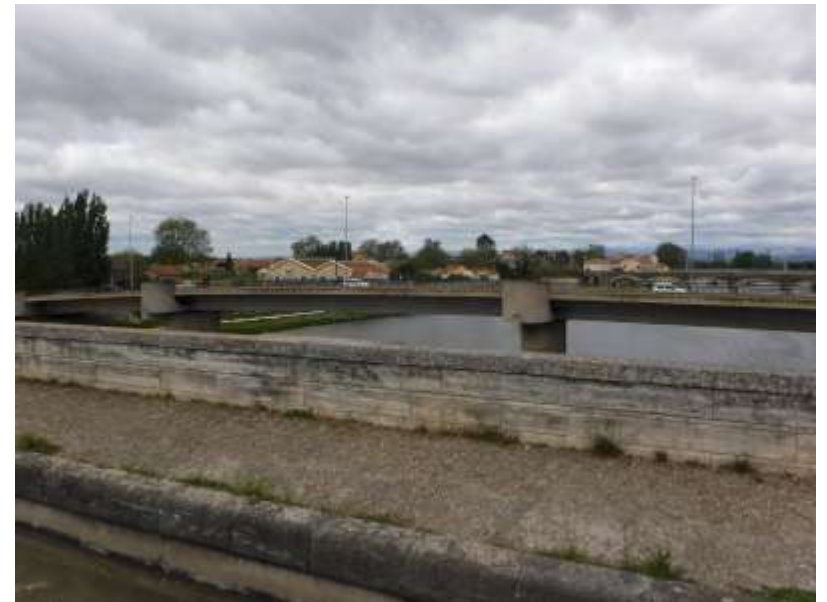
Aqueduct across the Orb River
